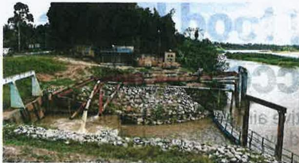
Water pumps are not as effective because of the high amount of sand and silt in the river.
