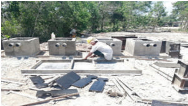
Precast Hydrant (Slab)
