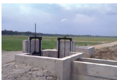
Struktur offtake line C2-C2A
