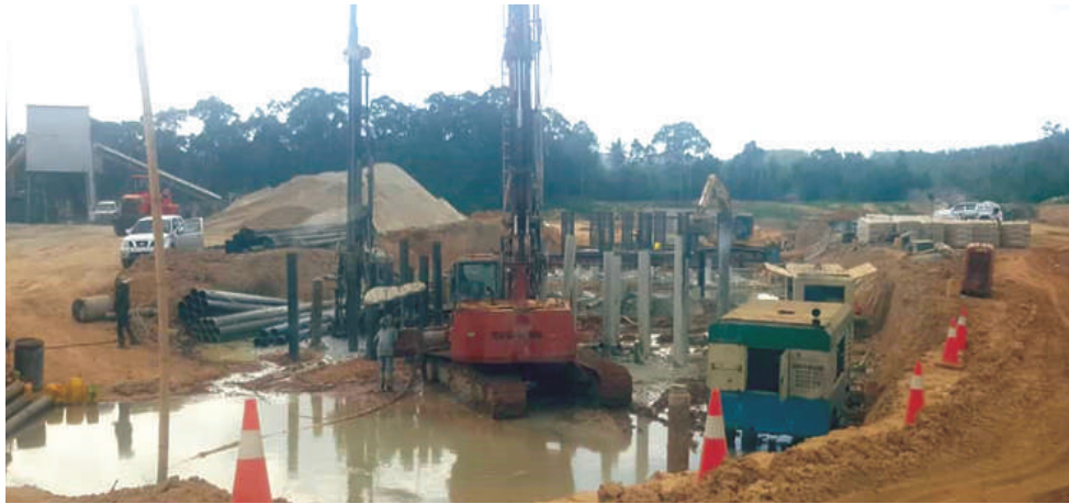
Figure 3Kerja – kerja micropile di Auxiliary Weir Bridge
