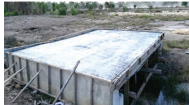
Concrete for Tractor Crossing
