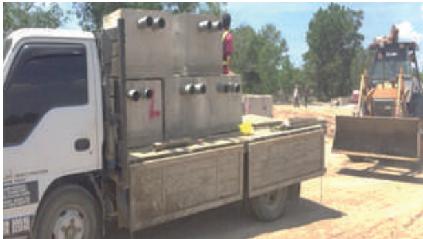
Transfer Hydrant to Site
