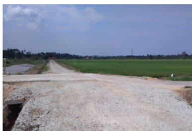
Rc approach road
