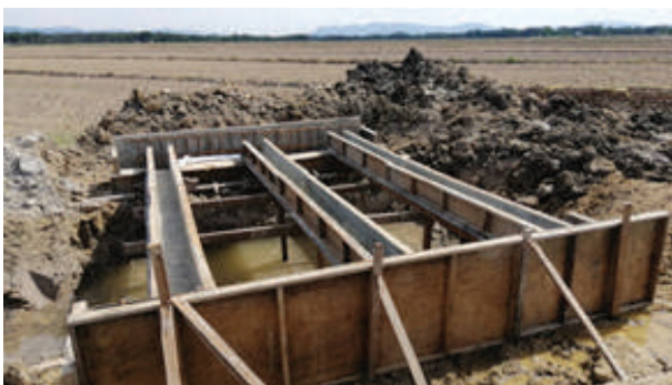
Formwork for Tractor Crossing
