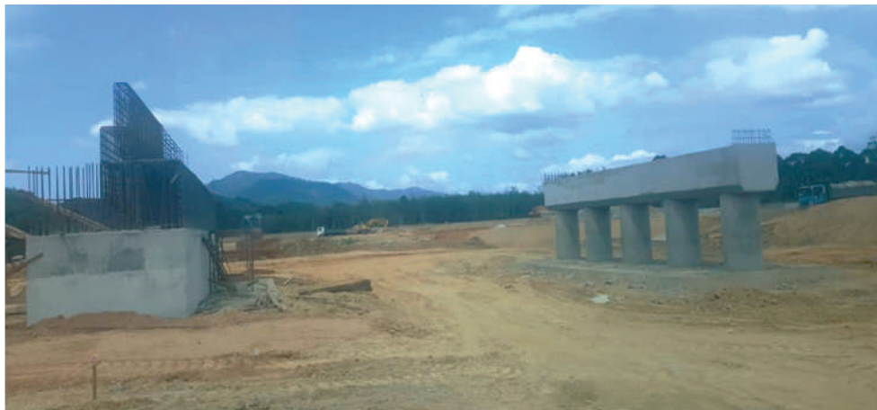
Abutment 1 dan Pier 1
