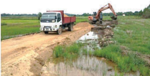
Farmroad Work (Lay Imported Soil – Second Layer)
