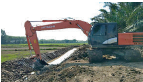
Drainage Work Type A
